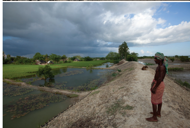
Figure 1a. Embankment ©hellio-vaningen 1b. Construction of embankment ©hellio-vaningen
